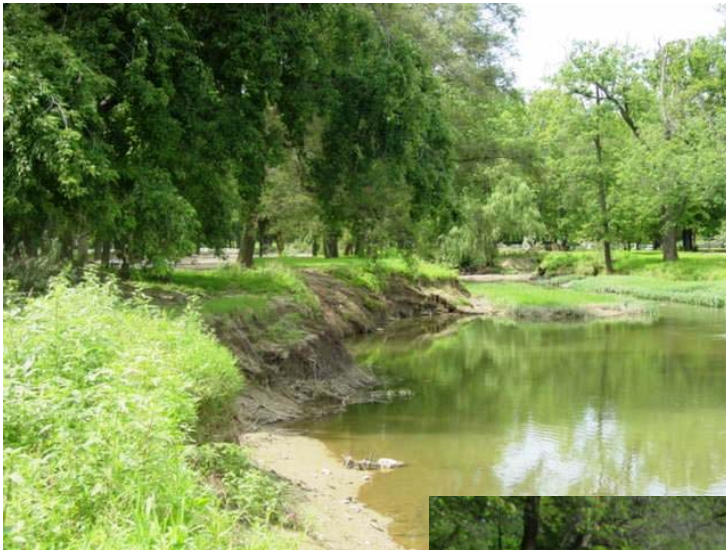
Left: Before construction. Highly eroded and unstable banks
